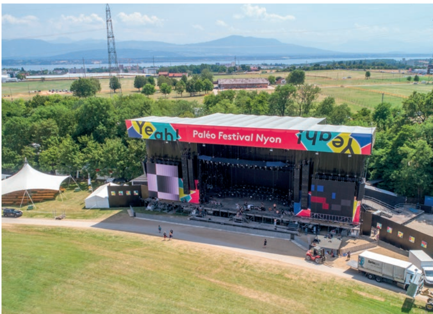
With a clear stage width of up to 31.4 meters, the Jumbo Stage offers an expansive show area.
