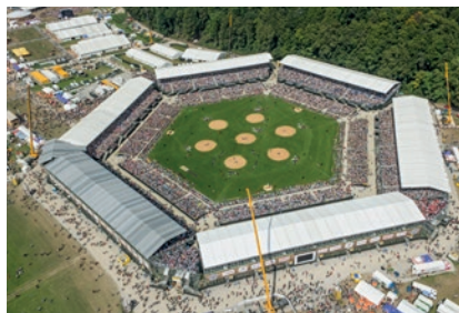
Modular construction on every scale, quickly built, safe, and spectacular
